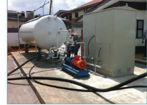
Skid Filling Plant With 5MT LPG Storage Tank
