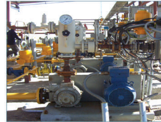
LPG Bulk Transfer Pumps and Pipeline Networks
