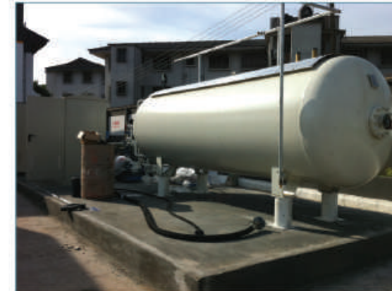
Skid Plant With 5MT Storage Tank Equipped With Fire Water Sprinklers
