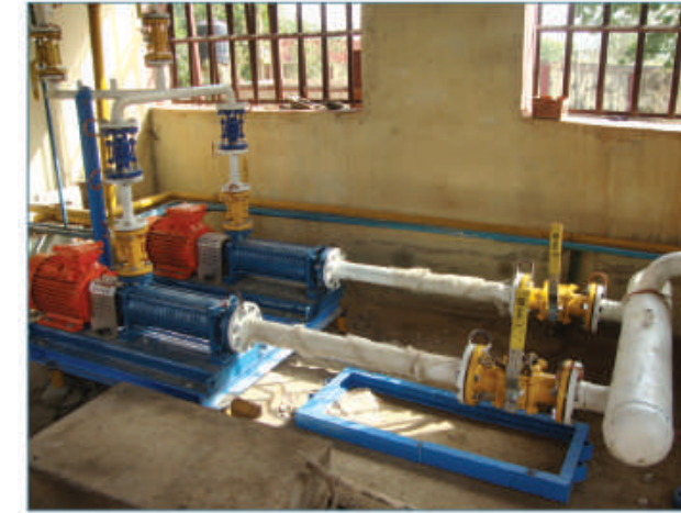
LPG Pumps & LPG Pumps House Piping Networks
